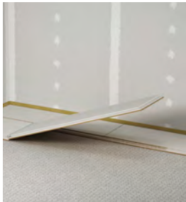
3. Install the fermacell flooring
