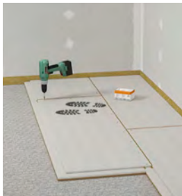
6. Fix by screwing or stapling within 10 minutes – stand on the overlapping edge element
