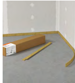
1 Fitting the perimeter strips
