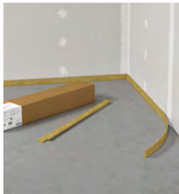
1. Apply perimeter strips and push into the perimeter junctions
